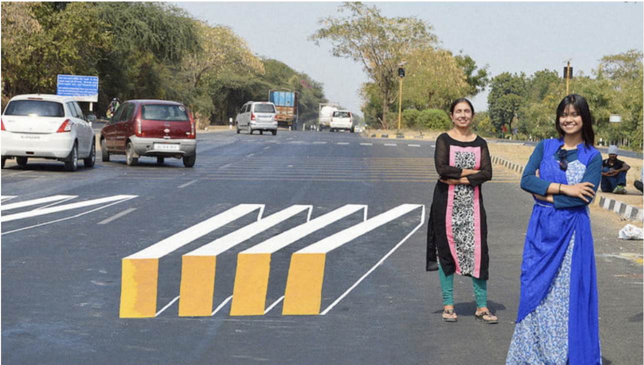
Figure 2: Optical illusion nudges for road safety in school zones in Ahmedabad, India
